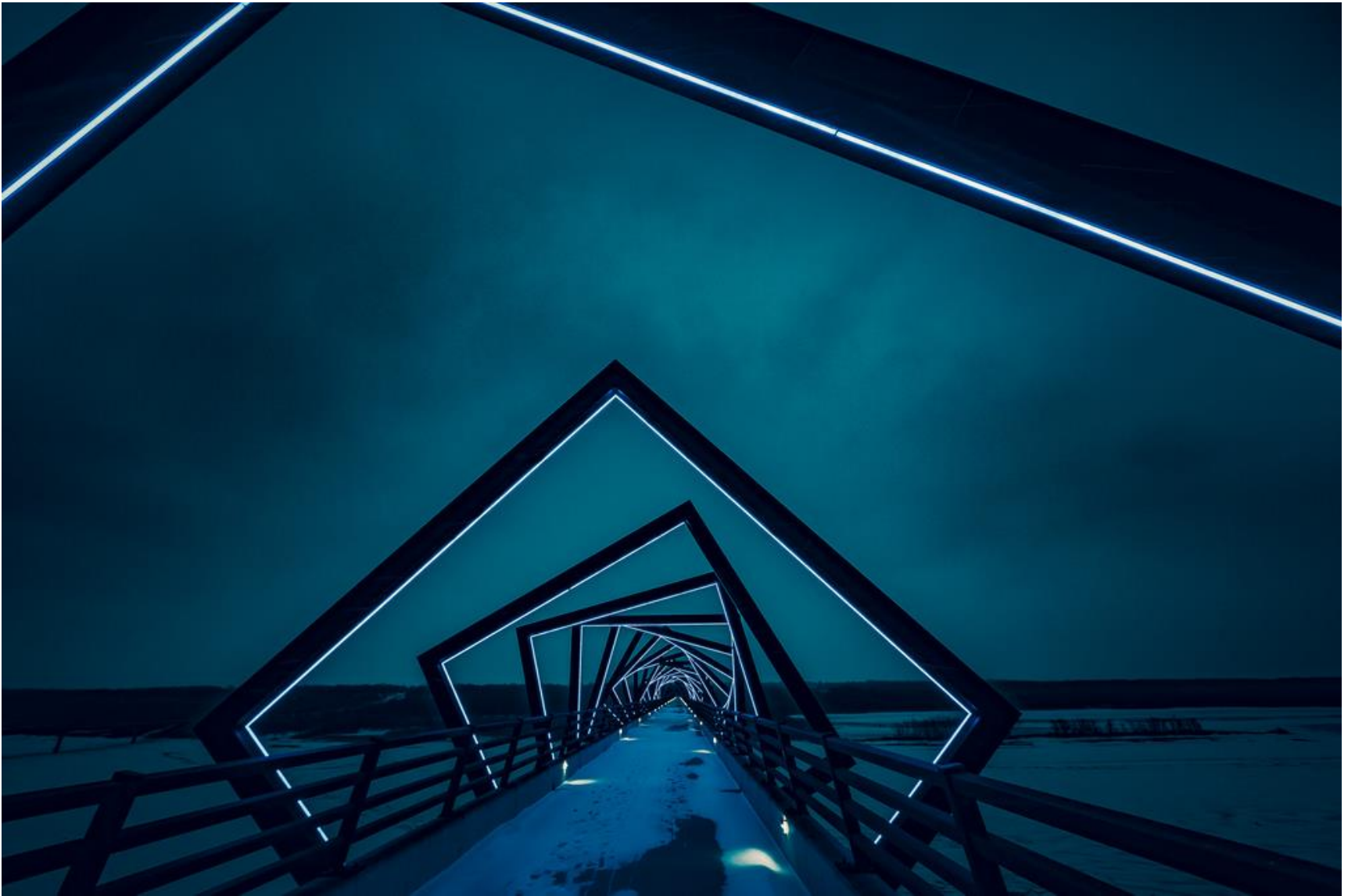
High Trestle Trail Bridge, Iowa. Photo by Tony Webster
